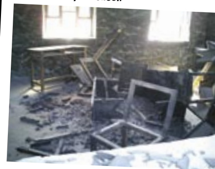
Taliban destroyed school.
